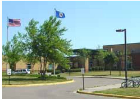
Hallberg recently performed recommissioning services at Skyview Community School in Oakdale.
